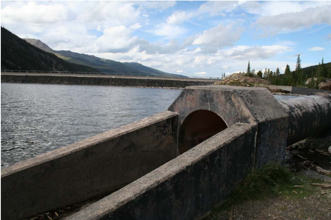
East Fork Conduit release into Homestake Reservoir, photo by James Heath
